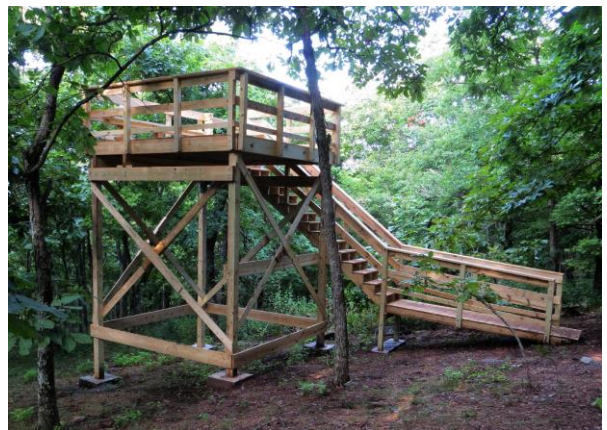
Completed South Tower
