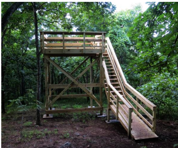
Completed South Tower
