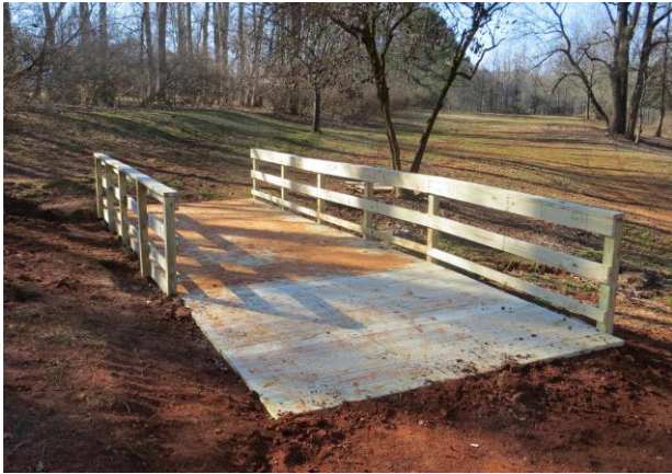
Bridge over Ravine
