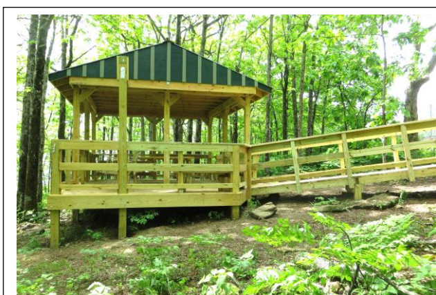
Pavilion with Handicap Ramp
